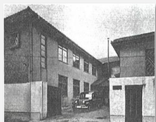
Factory and office in Oimatsu-cho, Osaka
