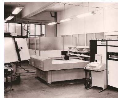
Grading machine modifies and cuts basic sewing patterns
